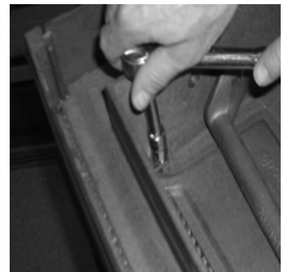
FIG. 17 Remove Damper Assembly
