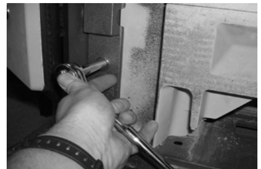
FIG. 8 Remove Lower Retainers
